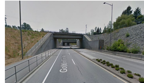
Figure 5: Intersection of Trans-Canada Highway and Golden Ears Way
