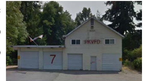
5. Port Kells Fire Hall No. 7
