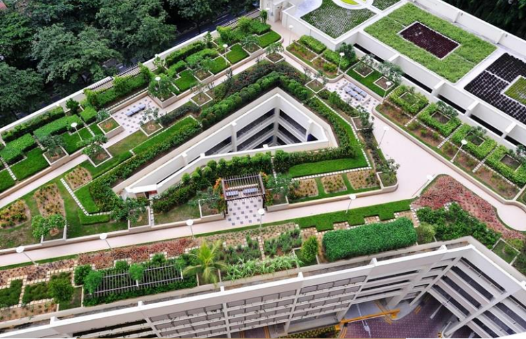
Photography of Roof Garden
