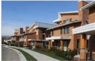
STREETSCAPE • TYPICAL LAYOUT ALLOWS FOR VIEWS TO MOUNTAINS FROM STREET • UNIFORM SCALE OF COURTYARD SINGLE FAMILY HOMES • SHARED ENTRANCE MANUVERS FOSTER COMMUNITY FEEL • INDIVIDUAL IDENTITY AT STREET ENTRY • NO LAKE ACCESS • MINIMAL COMMONLY SHARED SPACE • UNDERGROUND PARKING NOT ALWAYS FINANCIALLY VIABLE FOR SINGLE FAMILY IDENTITY • SIZE APPROXIMATE EQUIVALENT OF 4-60 LOTS COVERED
