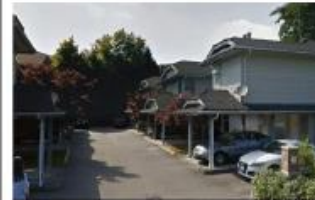
CENTRAL DRIVEWAY • TYPICAL HOUSING DESIGN IN HIGHWOOD, BC • APPROXIMATELY 1/3 OF LOT TAKEN UP BY VEHICULAR CIRCULATION • SMALL YEAR GARAGE, UNDESIRABLE NATURAL LIGHT • ALLOWS INDIVIDUAL IDENTITY OFF MAIN STREET • APPROXIMATELY EQUIVALENT TO 3 SINGLE FAMILY LOTS (FOUR-OR-THIRTSY) • ONLY "COMMUNITY SPACE" SIDE-HOLLAR CIRCULATION • NO BACK LAKE ACCESS • VEHICLE UNIT SIZES ALLOW FOR DIFFERENT FAMILY TYPES, SINGLES, COUPLES, FAMILIES, Etc.
